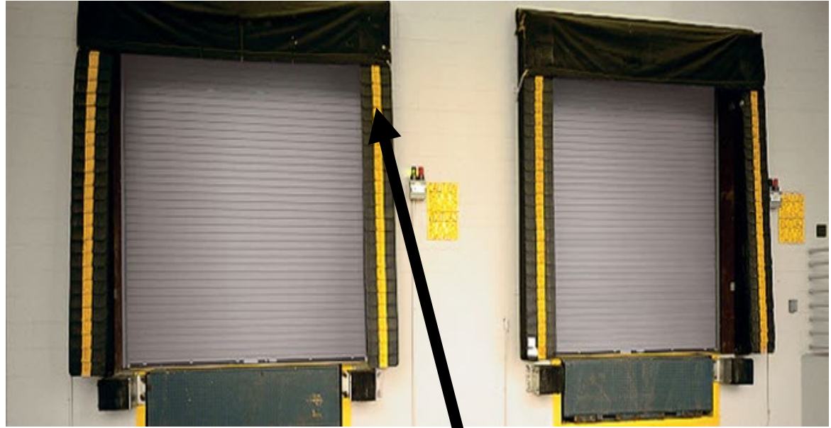
Damaged or missing pads
